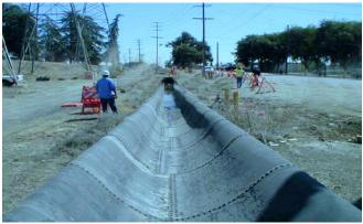
Vacuum: negative pressure in a pipeline causes it to implode and buckle in extreme conditions.
