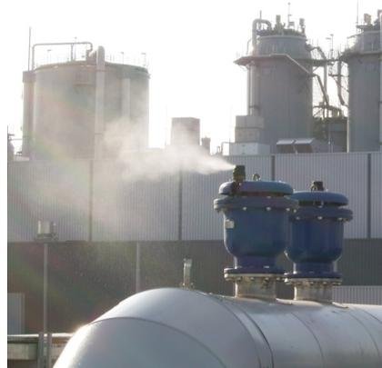
*Air entrainment; Air collecting at high points of the system reduces pump efficiency, causes corrosion and then as it is pressurised will create a small area of very high force, which can ultimately burst pipes.*
