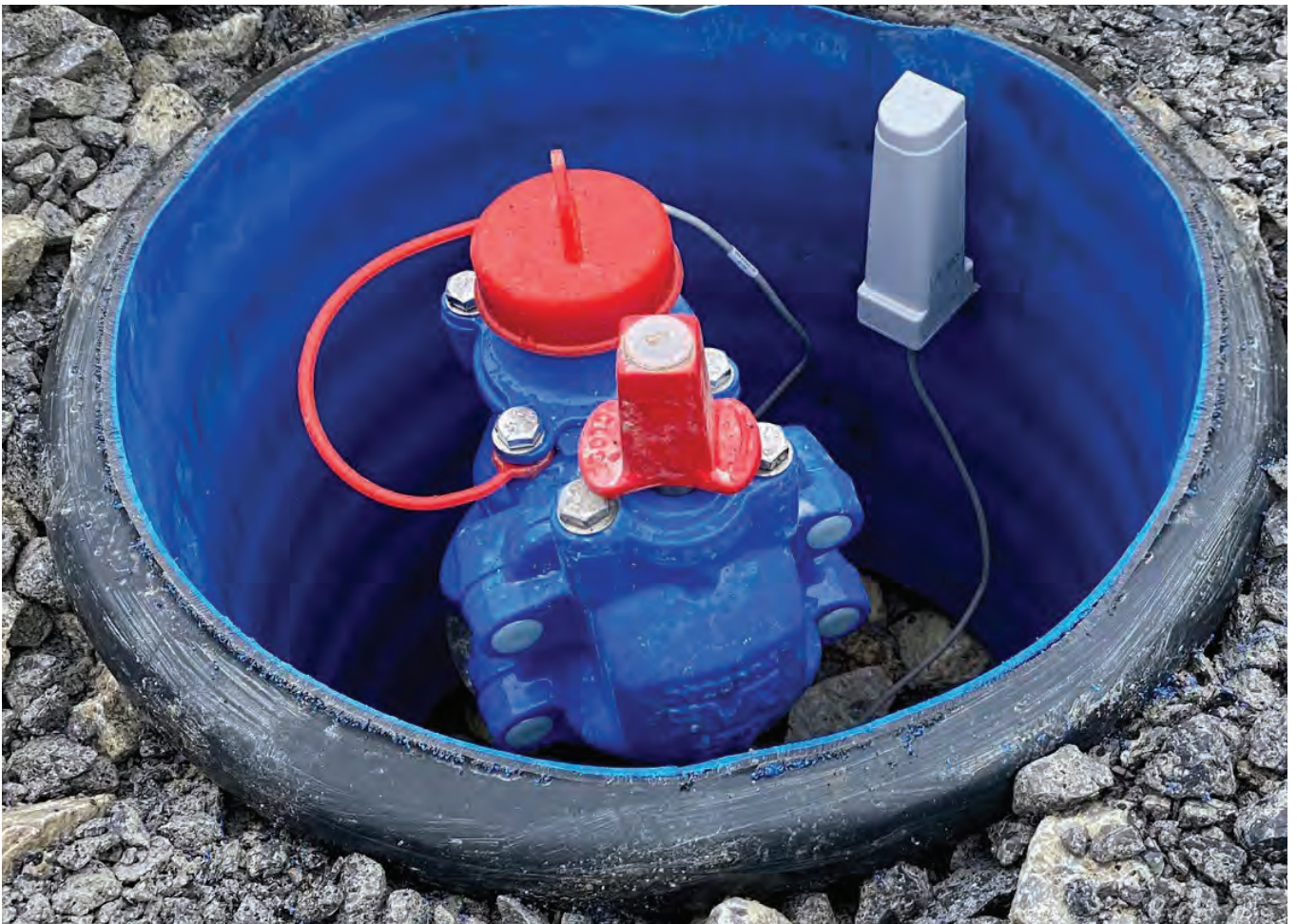
Hydrant with VIDI Temperature installed. VIDI Temperature is typically installed in combination with a gate valve, hydrant or similar. After installation, the device transmits information about the temperature in the network to the VIDI Cloud platform that stores the data.
